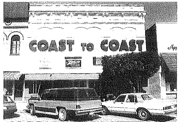
The second floor openings of this building have been inappropriately infilled with brick and an over-sized sign has been applied over this area. What was once a fine building with interesting brick detailing has suffered an almost complete loss of historic integrity.
