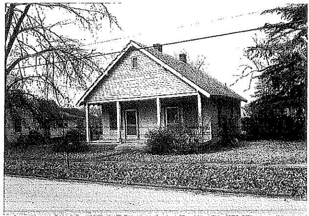
The integral or recessed porch is vital to the architectural integrity of the house type known as the Temple-front Cottage. The porch of this particular house has been well-maintained.
