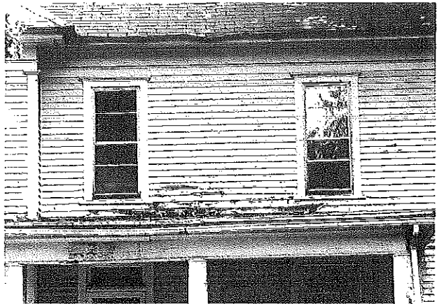
These replacement metal windows are inappropriate. A two-over-two pattern with horizontal muntins is not historically authentic, and neither is the metal material.
